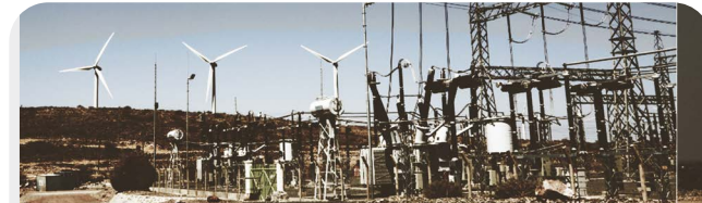
Reducing system Losses
